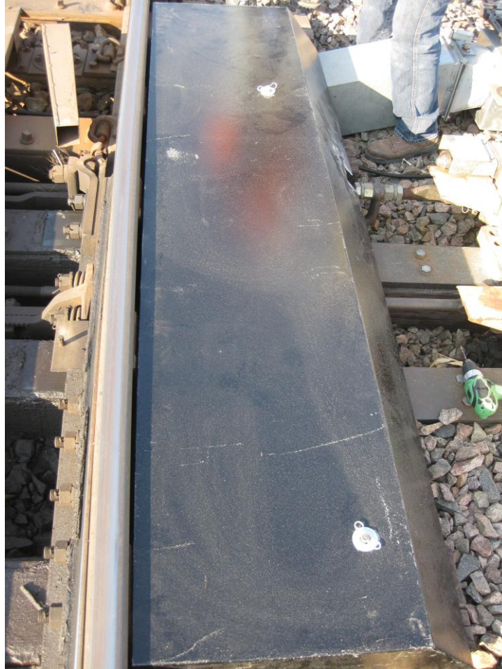
(Wide 8' Side Cover Installed)
