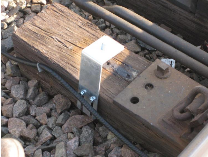
(Slotted Tie Bracket Installed)
